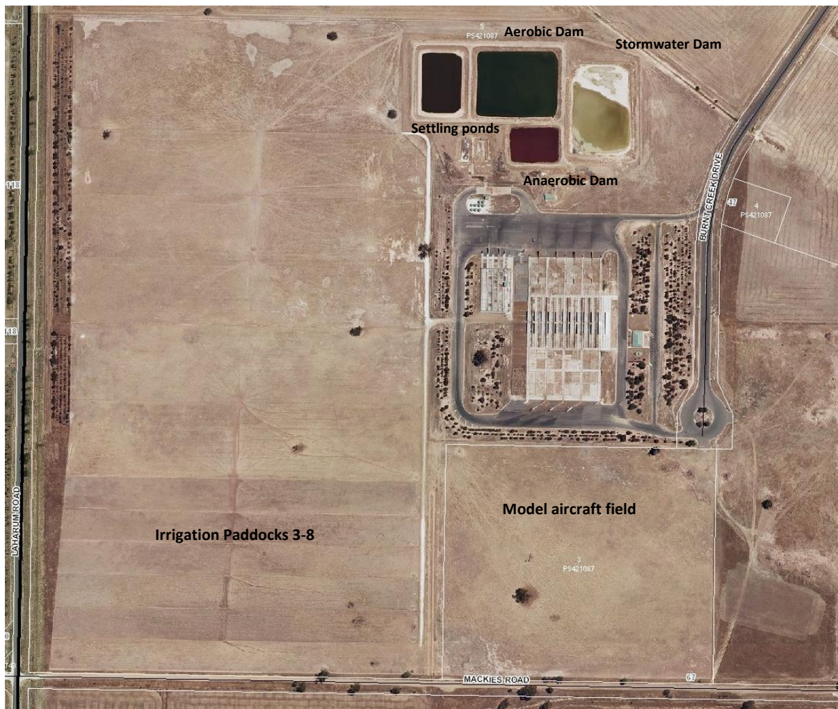
Figure 6: Aerial image of HRLE Site
