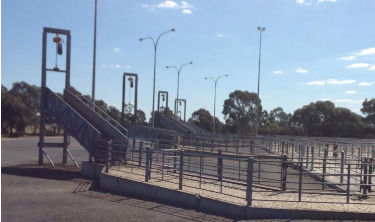
Out loading Ramps
