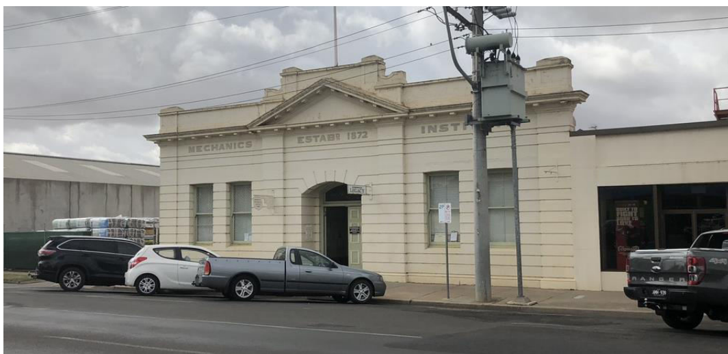
Premises of the Horsham Historical Society, Pynsent St, Horsham, January 2018
