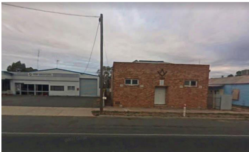
Premises of the Arapiles Historical Society, Natimuk, Horsham RC (image from Google Maps)
