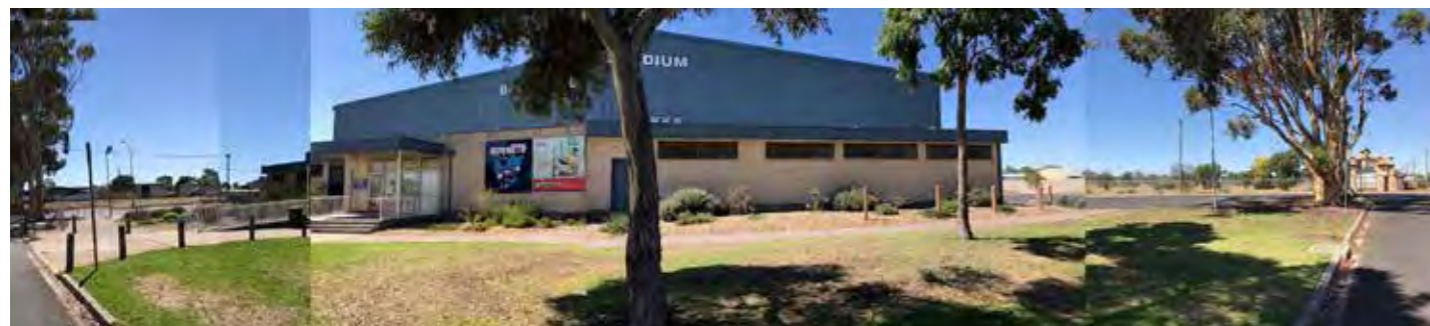
Existing McPherson Street Frontage
