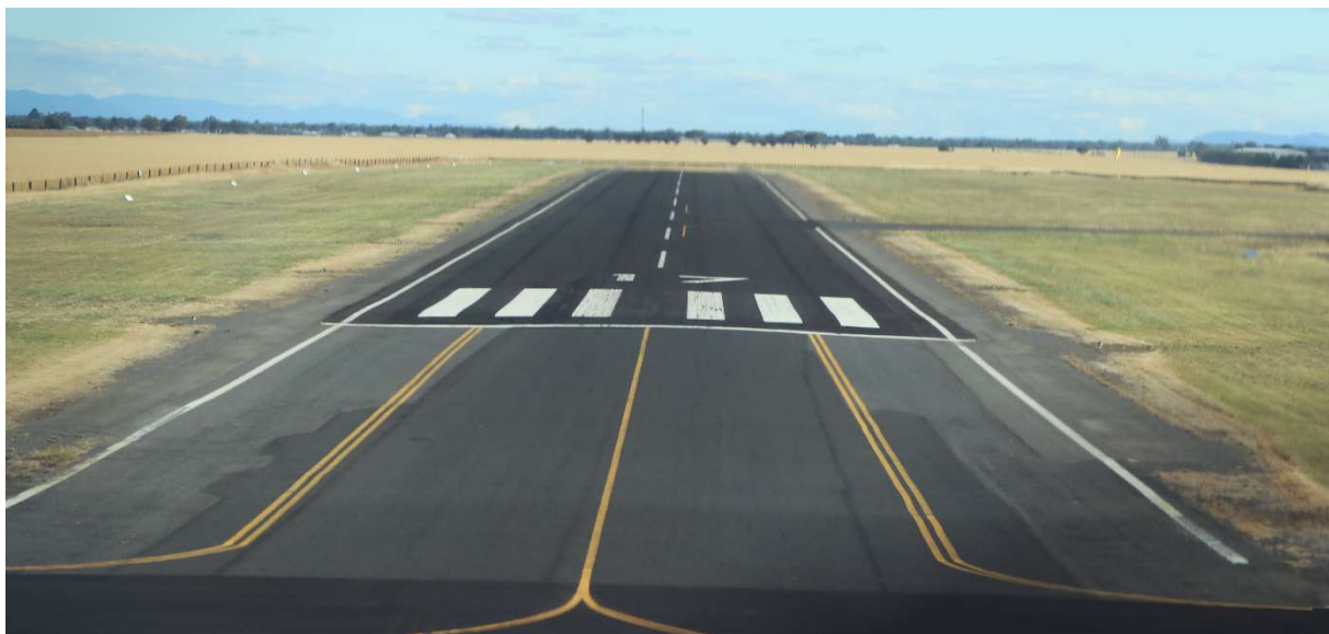
Source – HRCC JM - Horsham Aerodrome
