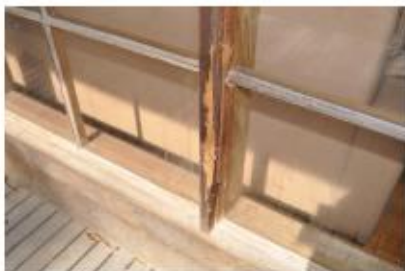
Figure 5: Cockatoo damage to timber window frames
