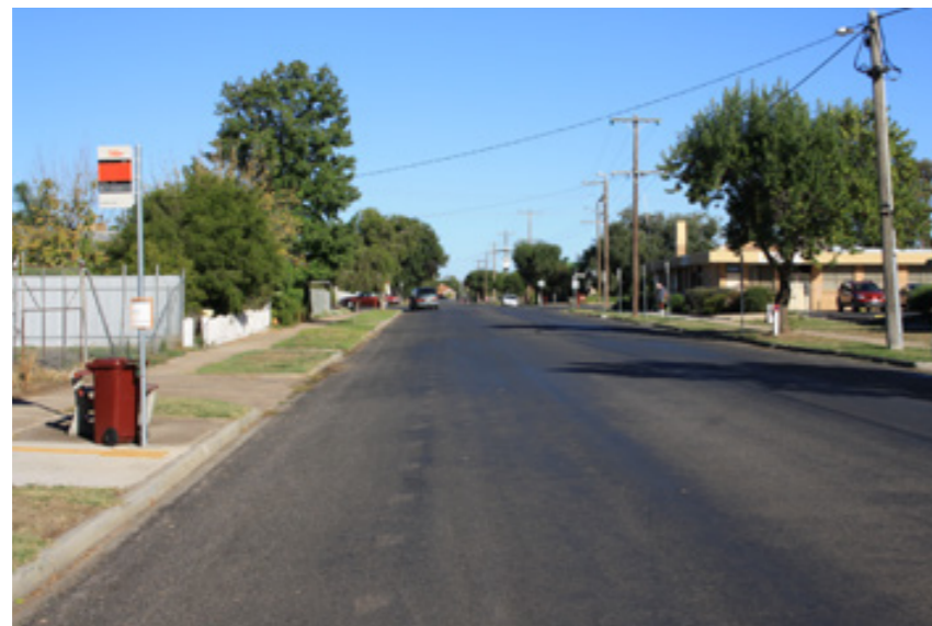
Existing conditions along Lynott St near level crossing
