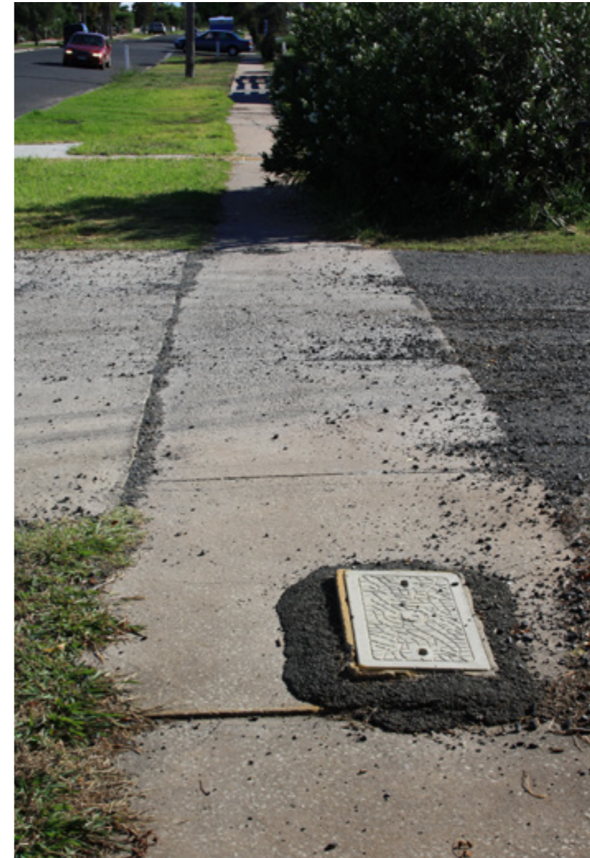
Example existing conditions
