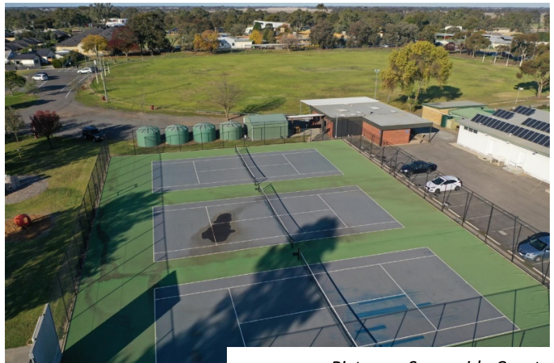
Picture – Sunnyside Courts Source – HRCC Drone
