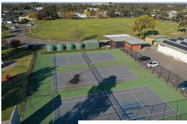
Picture – Sunnyside Courts Source – HRCC Drone
