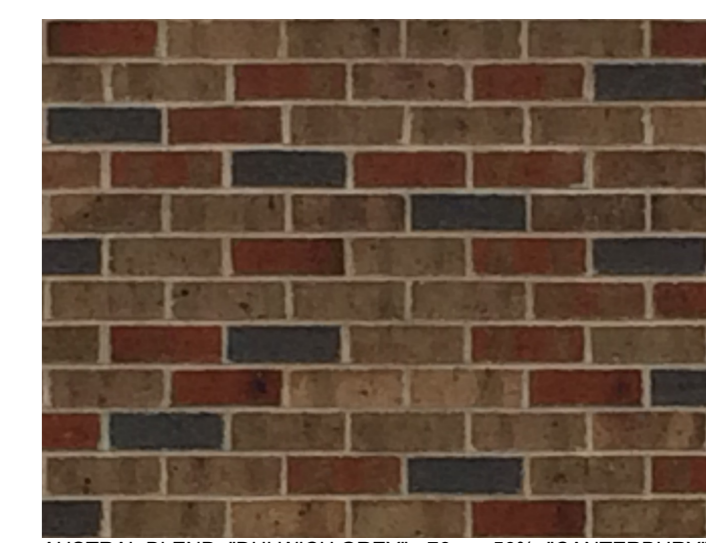
AUSTRAL BLEND: "DULWICH GREY" - 76mm 50%, "CANTERBURY" (RED) 30%, "ZINC WOLLERT" - 76mm 20%.
