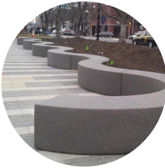
Insitu curved concrete seating
