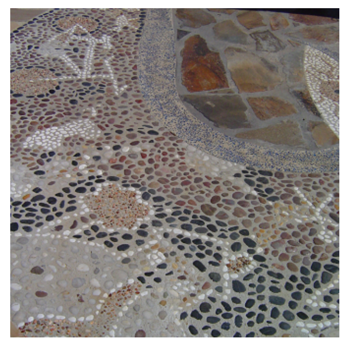
Mixed media paving
