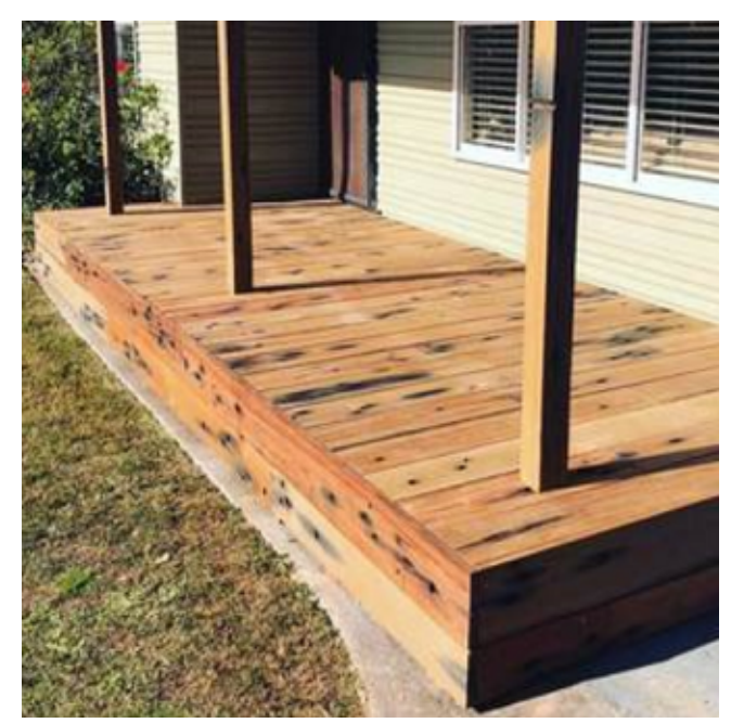
Reclaimed railway sleeper decking
