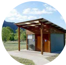
Toilet Block Landmark Coastal
