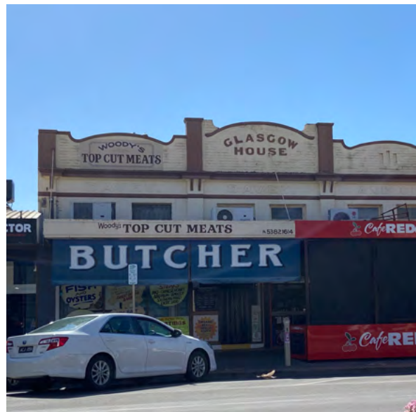
There are a number of beautiful parapets throughout the town that are candidates for restoration
