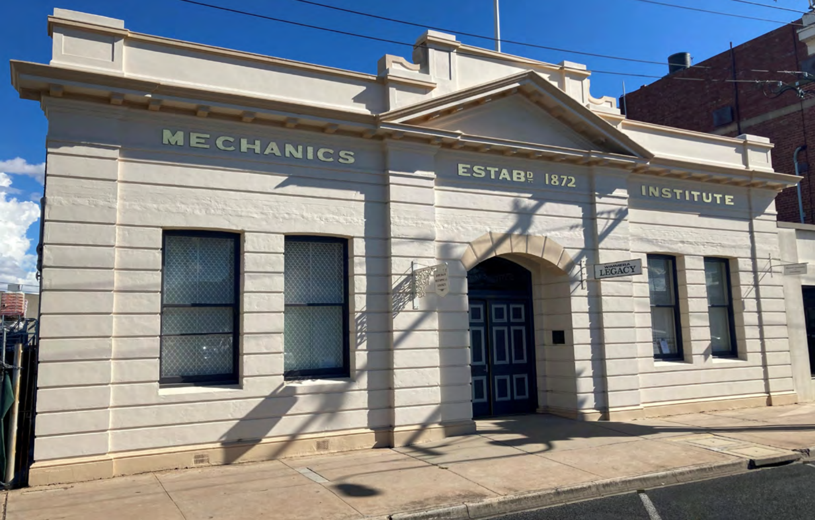
Freshly painted Mechanics Institute on Pynsent Street is an excellent example of appropriate heritage improvements
