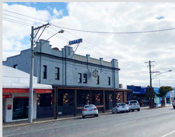
The Bull and Mouth is one of the heritage buildings on Wilson Street. Currently there is no streetscape amenity on this part of the street.
