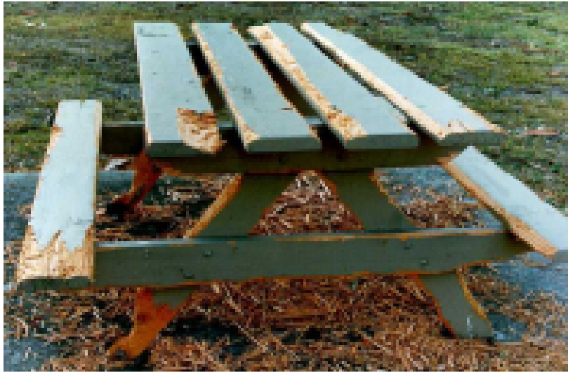
Figure 6: Cockatoo damage to outdoor furniture
