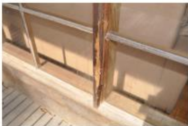
Figure 5: Cockatoo damage to timber window frames
