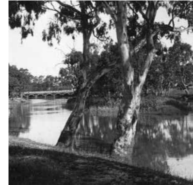
Western Highway bridge over the Wimmera River, Horsham, 1930. Image: HHS 010994
