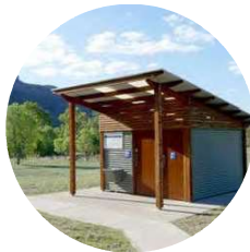
Toilet Block Landmark Coastal
