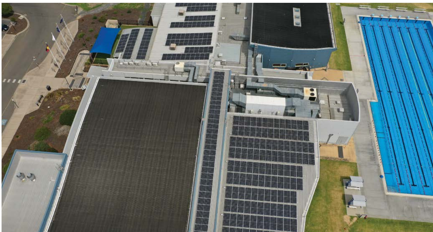
Solar panels were installed on the roof of the Horsham Aquatic Centre and several other Council buildings this year (page 55)
