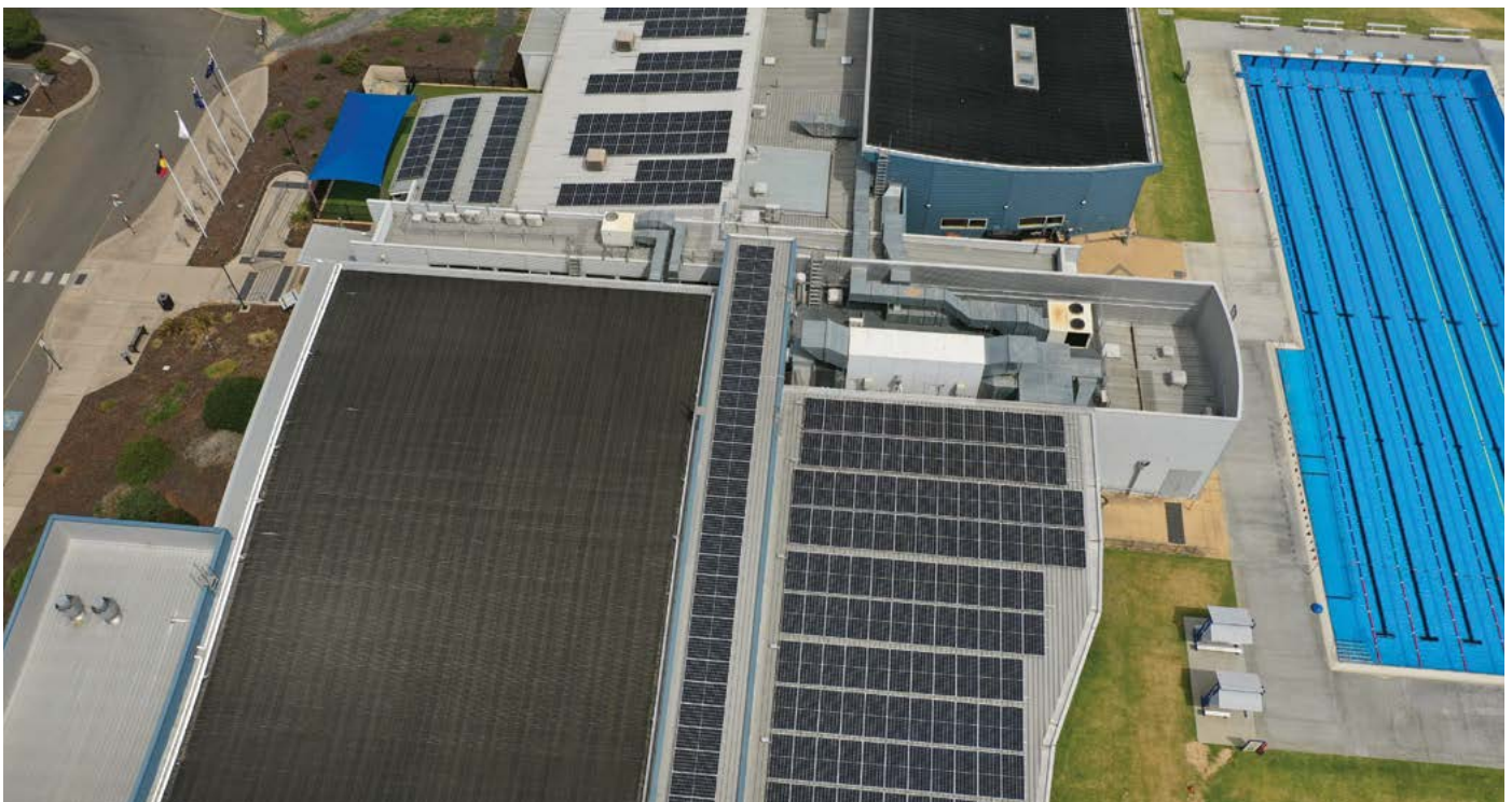
Solar panels were installed on the roof of the Horsham Aquatic Centre and several other Council buildings this year (page 55)
