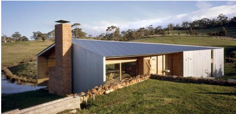
Image 4: A contemporary interpretation of a rural working shed (Design by John Wardle Architects)
