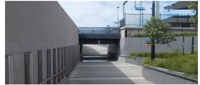
Cardinia Road underpass, Pakenham (Department of Transport and Planning)
