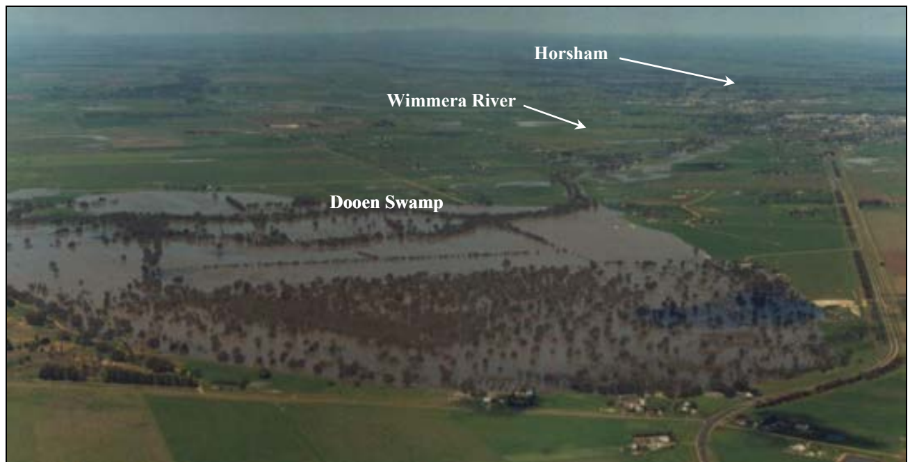
Figure 2-7 Aerial View of Dooen Swamp – 1988 Event (Provided by Wimmera CMA)
