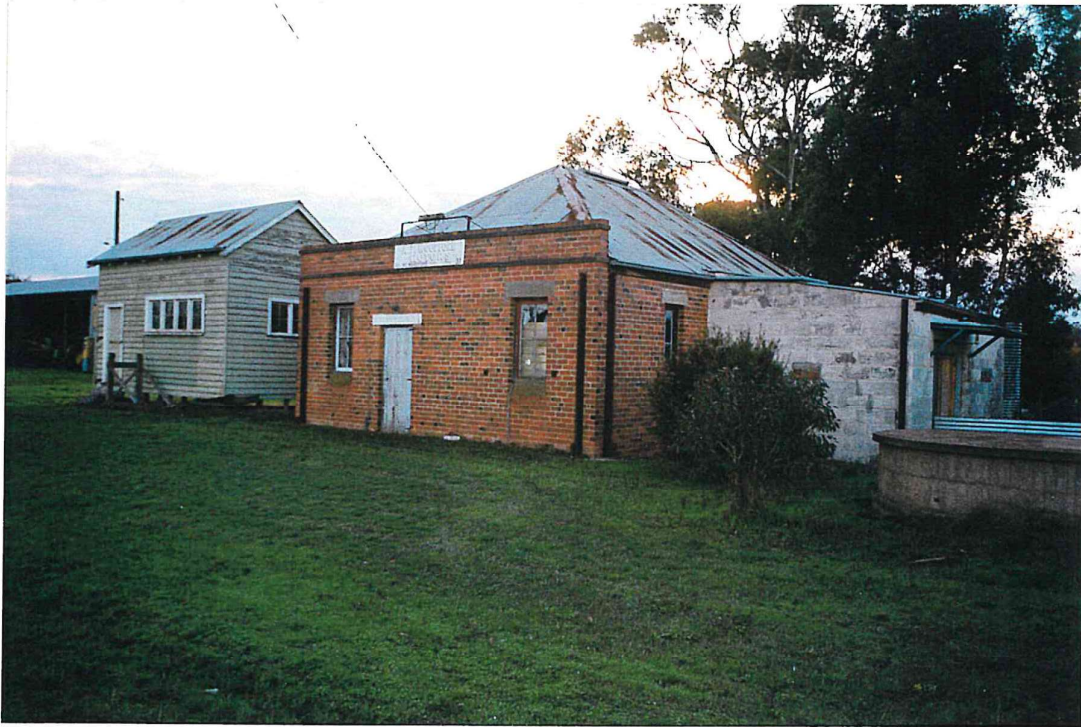
Newton and Millers' office and the former powerhouse
