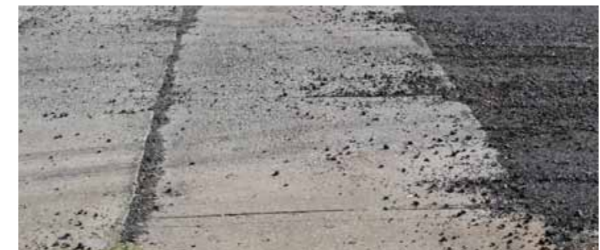
Example existing conditions
