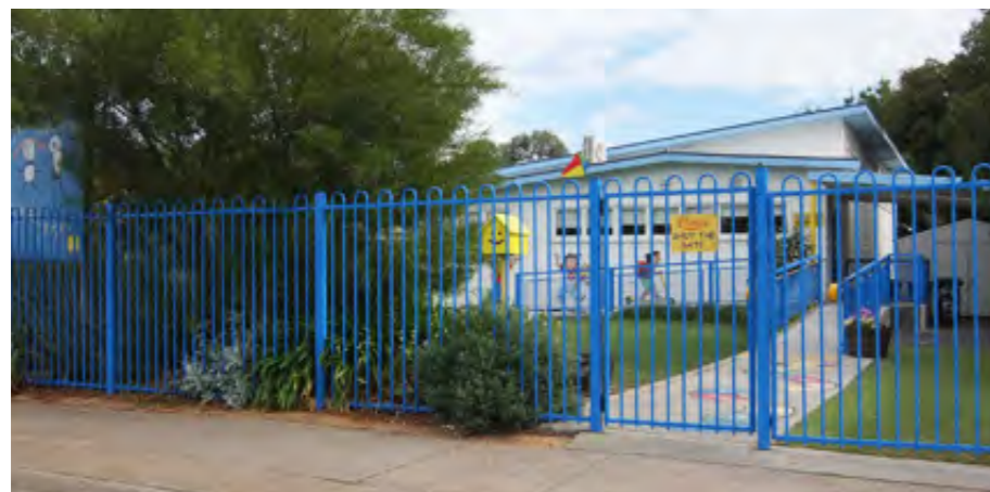
View of Entry Gate from Natimuk Road
