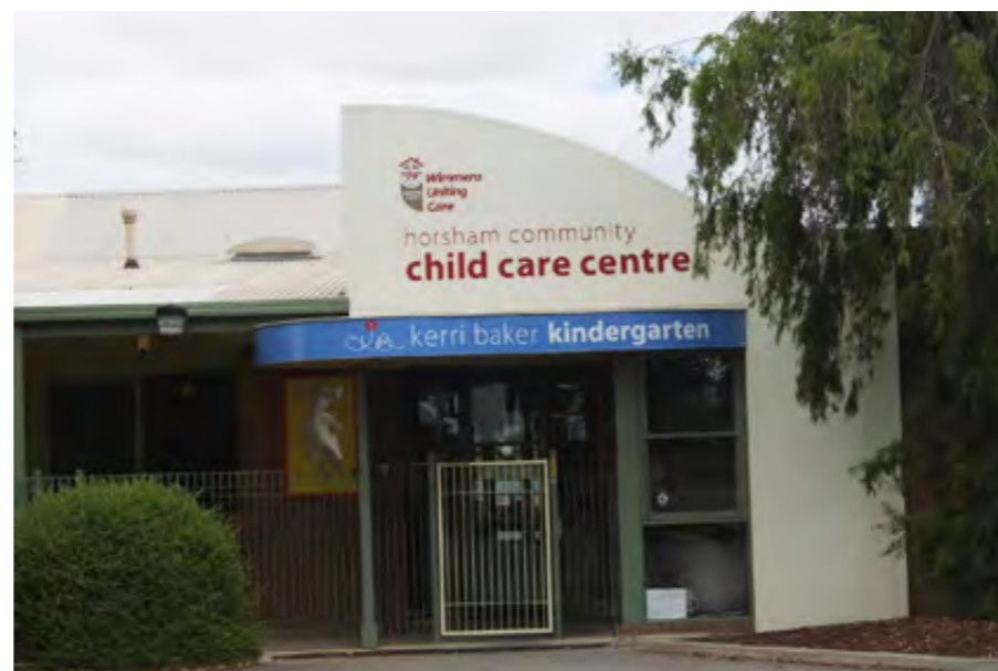
View of front Entry
