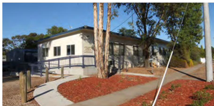
Robin Street view of Kindergarten & MCH Building
