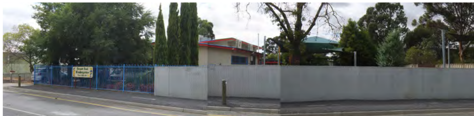
View from Bennett Road corner
