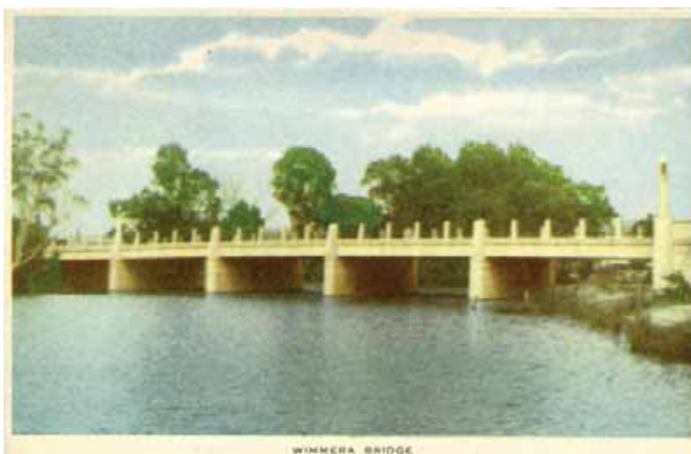
15.2 The new Bridge over the Wimmera River, completed in 1939 (State Library of Victoria)
