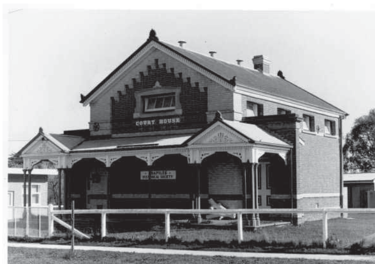
10.1 Natimuk Court House, photographed in 1970 by John Collins (State Library of Victoria)
