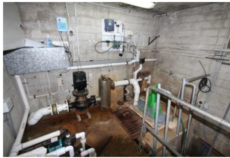
Original Filter & Pump room (still in use)
