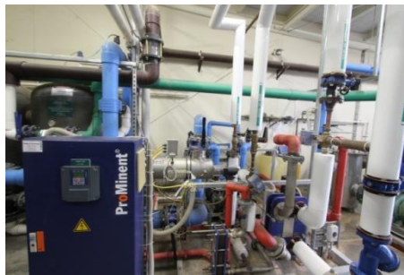
Existing Pump room (25m & Leisure Pools)
