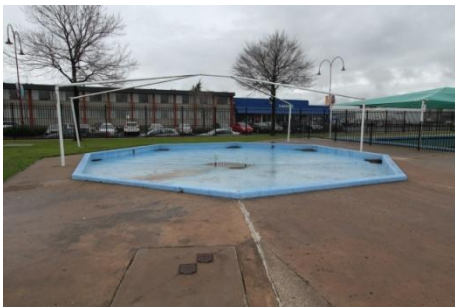
Existing toddler pool (Cracked)
