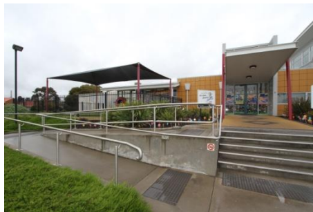
Existing Entry – Ramp requires upgrade
