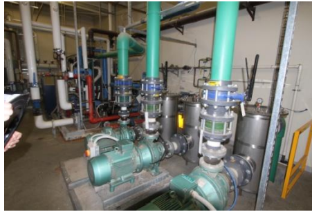
Existing Pump room (25m & Leisure Pools)
