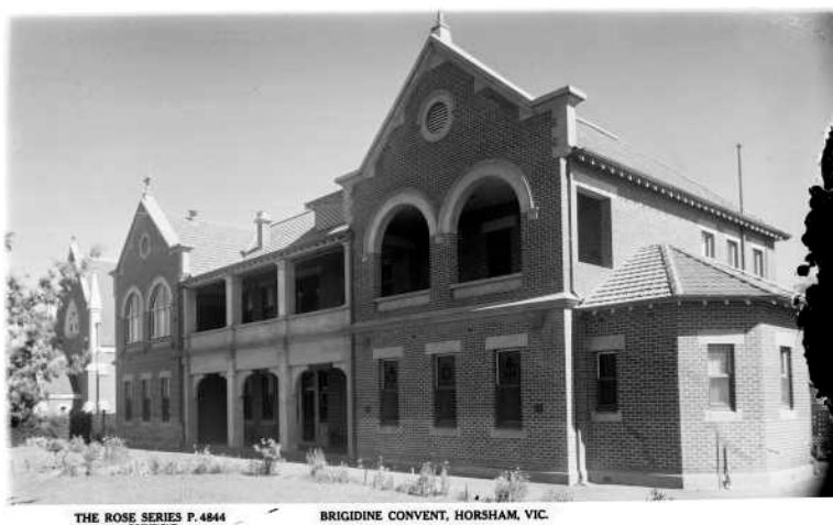
24.2 Brigidine Convent, Horsham, opened in 1920 – now demolished (State Library of Victoria)
