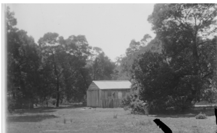
11.1 Timber bee-keeper's hut belonging to Matthew Matthews at Bald Hills, Laharum (State Library of Victoria)
