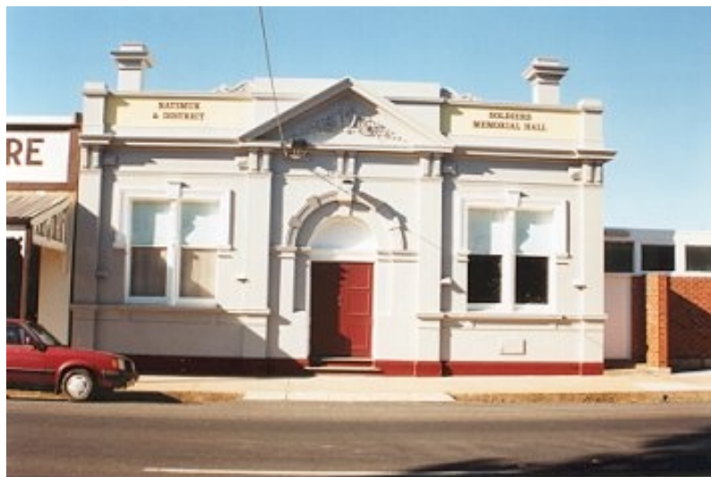
25.1 Natimuk Memorial Hall erected in 1909 (National Trust of Australia)
