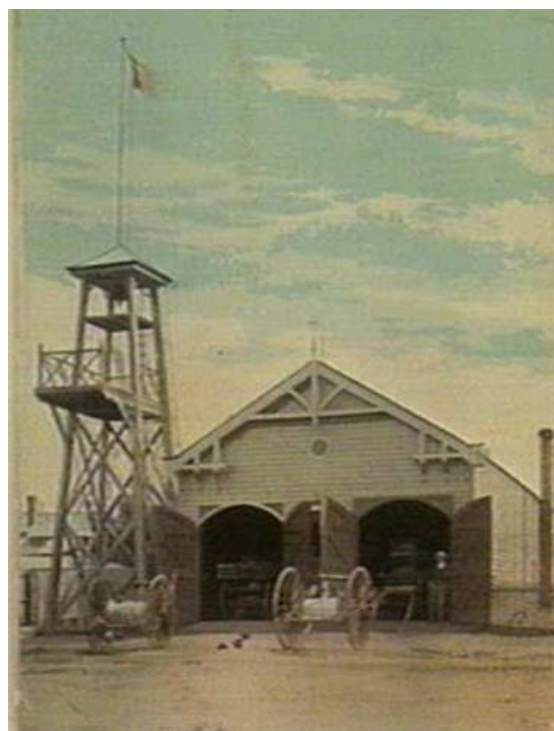
22.2 Horsham Fire Brigade station and fire tower, c.1900s (State Library of Victoria)
