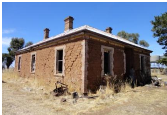
Oakville Park, Vectis c1900 mud brick homestead (2014)
