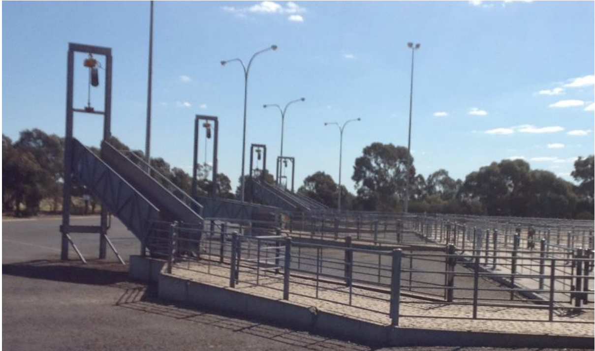
Out loading Ramps
