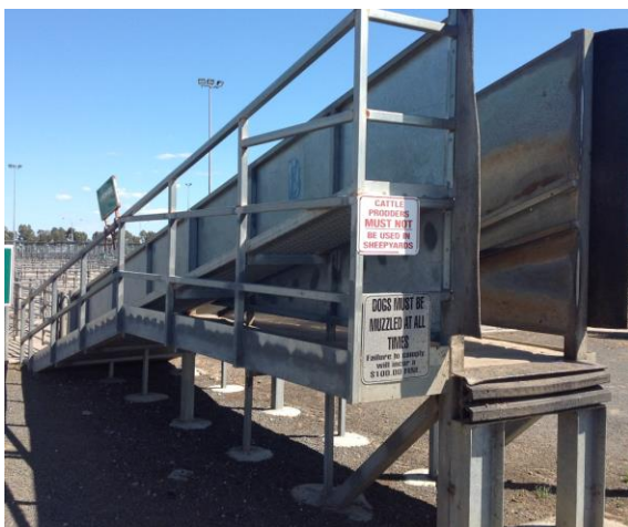
Remaining 2 Deck Loading Ramp to be replaced
