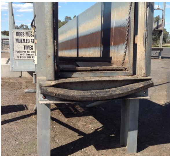
Buffer damage
