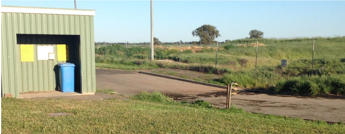
Truck wash and pump shed
