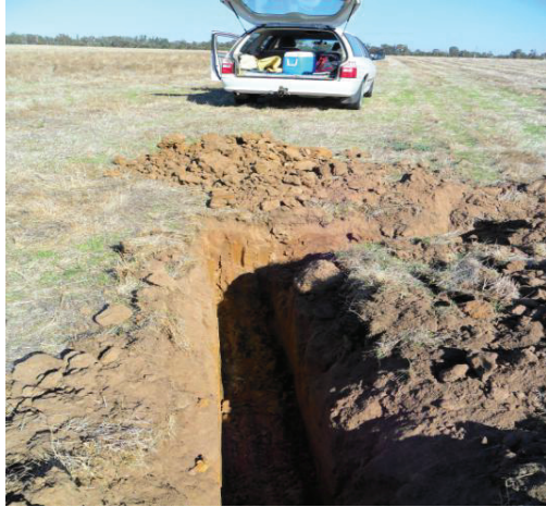
Lot 1 Soil Test Category 5 Clay soil at 150mm
