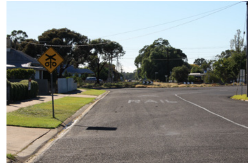
Existing conditions along Edith St near level crossing
