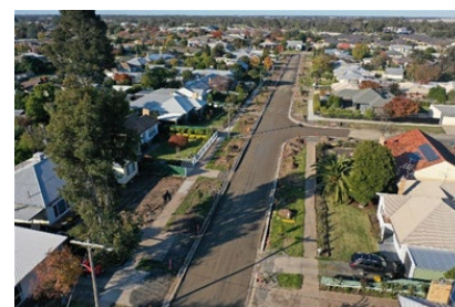
Picture – Johnson St Horsham works in progress 2019-20 Source HRCC Drone
