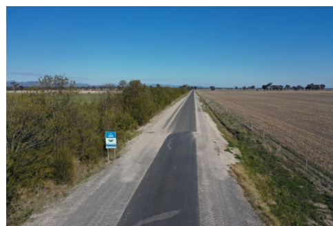
Picture – Green lake Rd after reconstruction in 2019-20 Source – HRCC Drone
