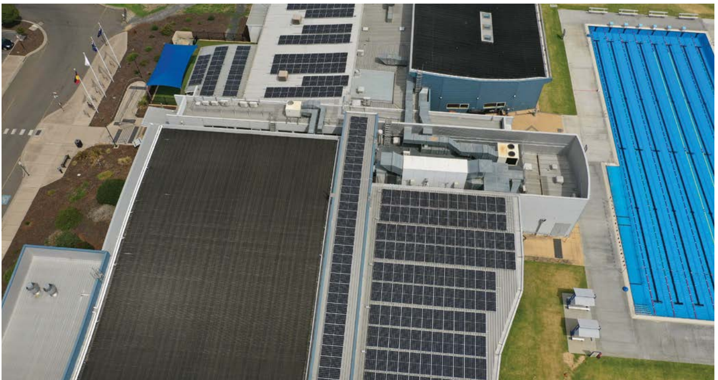
Solar panels were installed on the roof of the Horsham Aquatic Centre and several other Council buildings this year (page 55)
