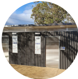
Toilet Block Exloo
