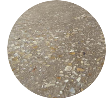
Exposed aggregate concrete coloured paving
