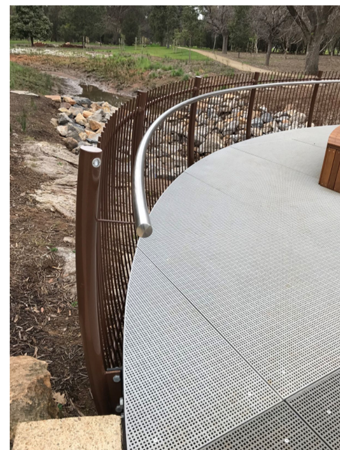
Inspirational Photo: Micromesh decking with handrail. Proposed design to have a double handrail and no gap between infill and decking
