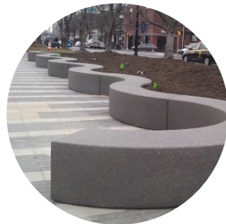
Insitu curved concrete seating
