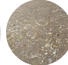
Exposed aggregate concrete coloured paving
