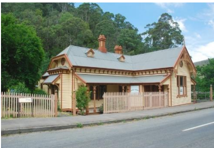
Former Walhalla Post Office and Residence Walhalla Walhalla Board of Management
