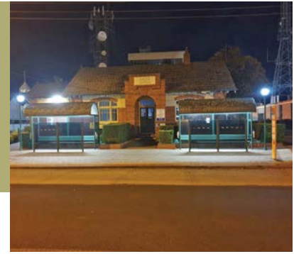
Additional lights were installed at the Roberts Avenue carpark this year.
