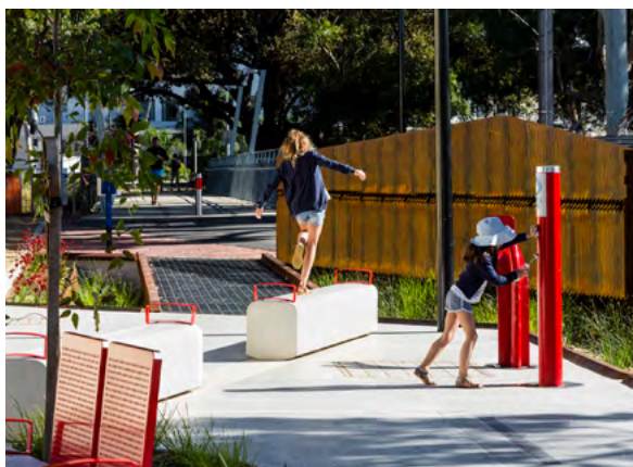
A shared street with flush kerbs demarcating space
