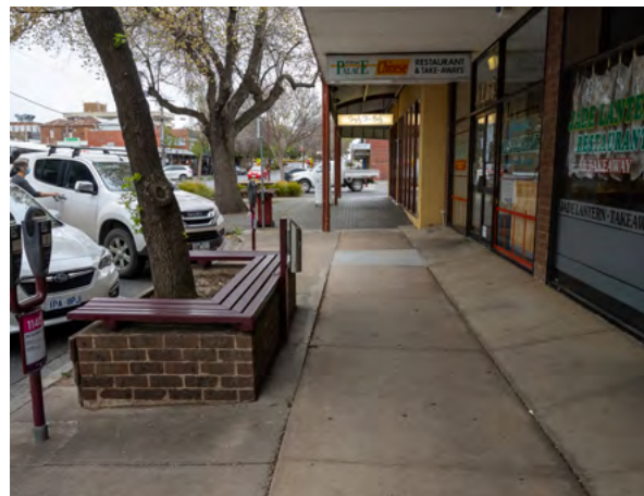
Tired street furniture should be updated and modernised. Additionally awkward grade changes should be assessed as part of a DDA and universal access study.
