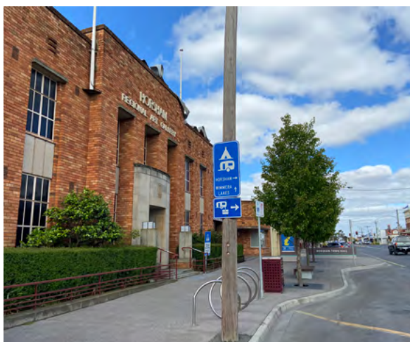
The Horsham Regional Art Gallery triggered some minor streetscape improvements including kerb out-stands, street trees and bike racks. It suggests how the entire street could be improved.
