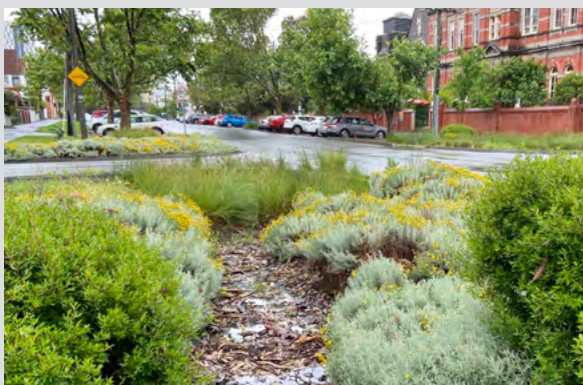
Stormwater management area in kerb out-stands at an intersection
