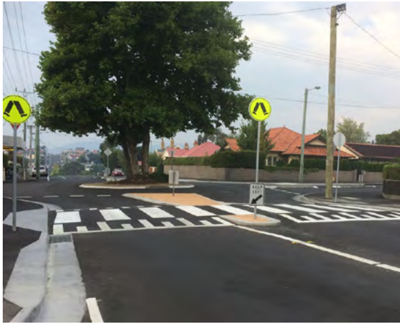
A raised wombat crossing designed to provide safe passage for pedestrians.
