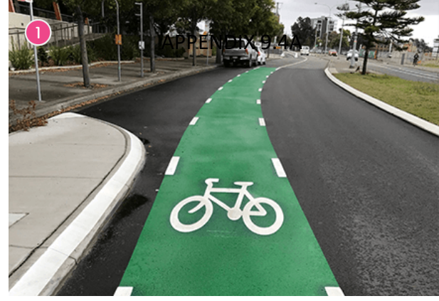
Addition of bike lane between parallel parking and carriageway still leaves plenty of room for vehicles to manoeuvre
