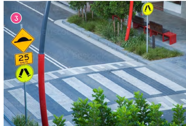
Mid block crossing with planting increases safety for those crossing at Gleed Street, and adds amenity to the street
