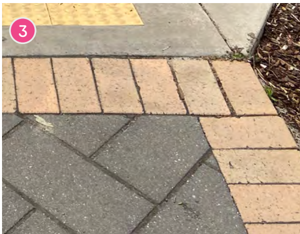
Warm Stone / Biscuit Blend Soldier Course Supplier: UrbanPave or equivalent Use: Edging for footpaths
