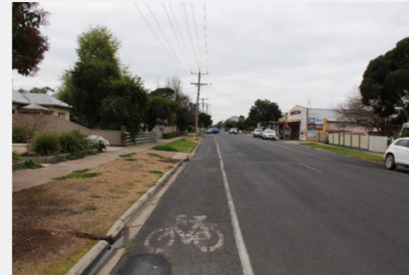
Bennett Rd looking north – Cycle lane on western side of road. Different width to lane on eastern side of the road.
