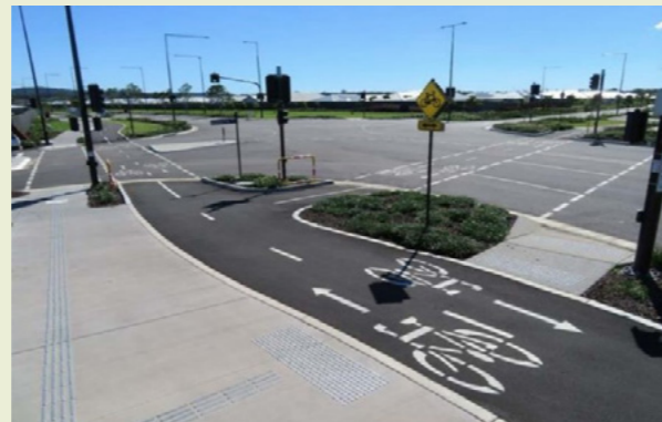
Treatment creating a protected intersection. Note the continuous cycle path and separation from pedestrians. Note also the landscaping barrier between vehicles and bicycles.
