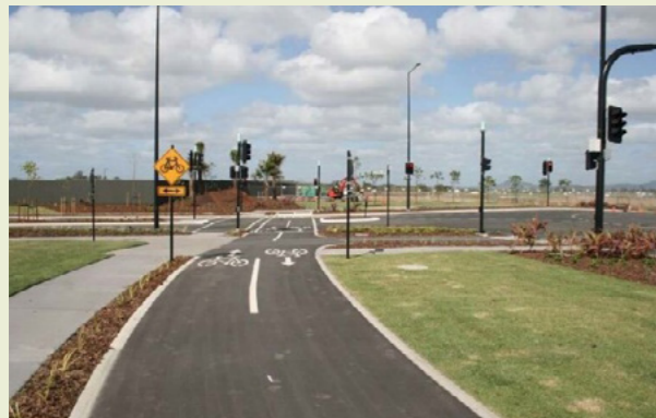
Two way cycle lane with line marking to provide colour contrast.
