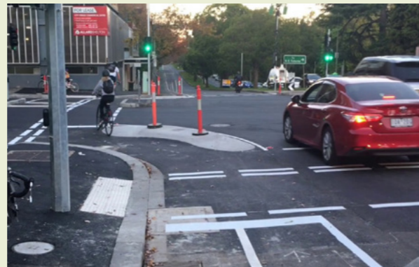
Protected intersection – Cyclists are separated from traffic. The 'jellybean' safety island increases sight lines for vehicles turning left.
