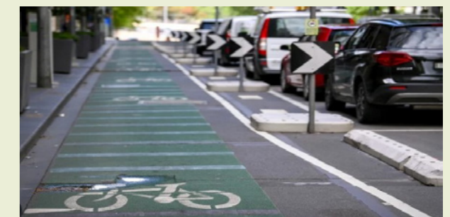
Protected cycle lane – Physical barrier and signage separates cycling from other road use.
