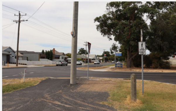
Baillie St – Park Drive intersection.
