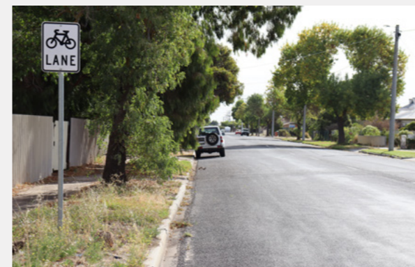
Lynott St (near Albert St intersection) – Faded line marking and car parked in cycling lane.
