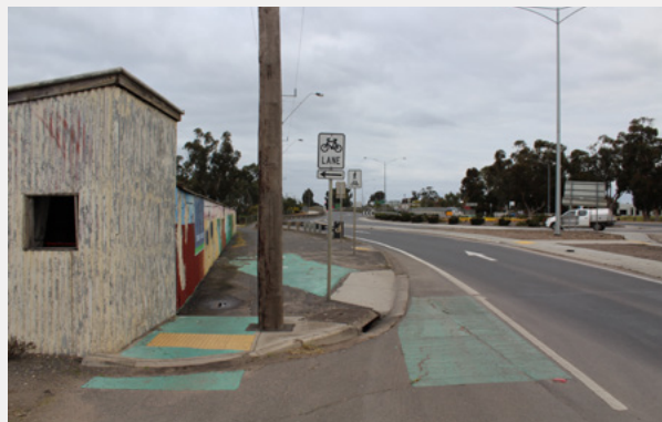
McPherson St near Stawell Rd intersection – Unprotected cycle access to off-road (shared) path. Kerb treatment not consistent with preferred cycle treatment.
