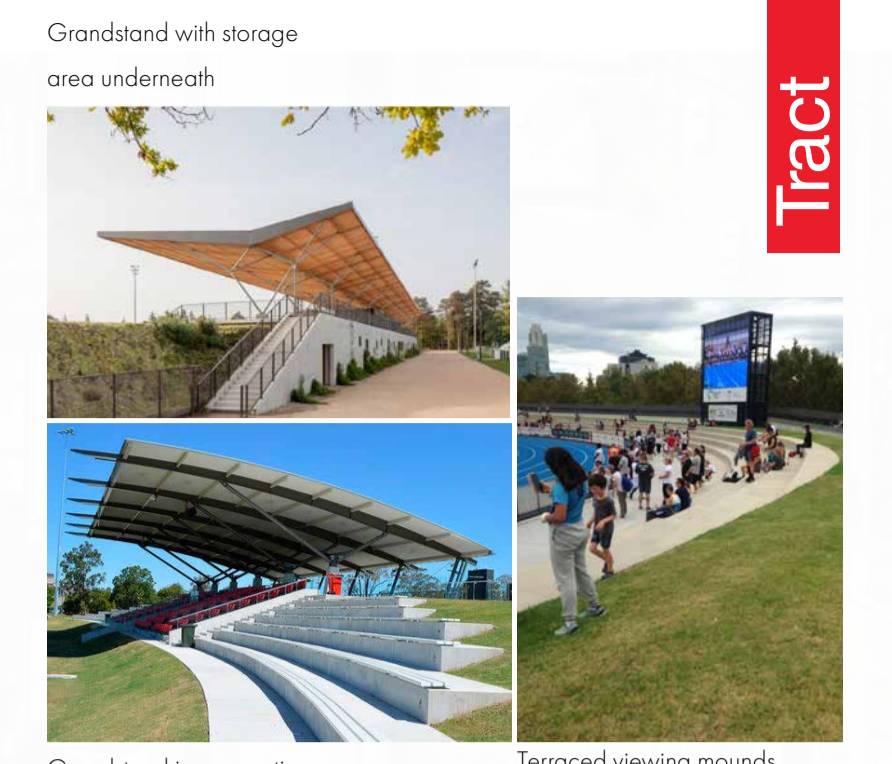
Grandstand with storage area underneath Grandstand incorporating terraced seating Terraced viewing mounds incorporating ramped access
