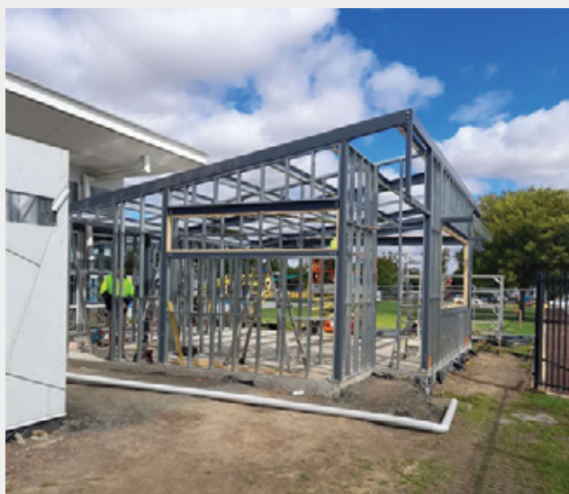
Aquatic Centre frameworks for change rooms.
