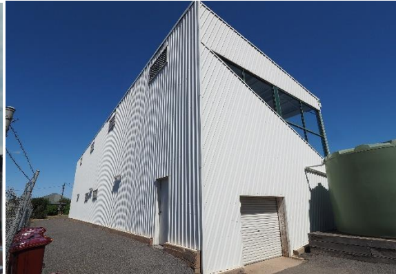
Figure 10: metal cladding installed
