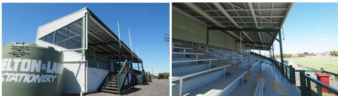
Figure 4, 5: Views of Horsham Grandstand (courtesy Stephanie Harder, Horsham Rural City Council)
