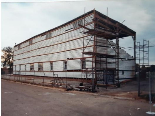
Figure 9: Grandstand prior to recladding:
