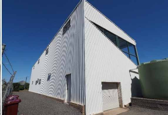
Figure 10: metal cladding installed
