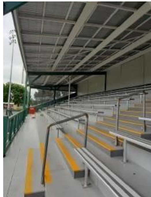
Figures 13, 14: Earlier timber seating and floor finishes, replaced with aluminium bench seats, floors covered
