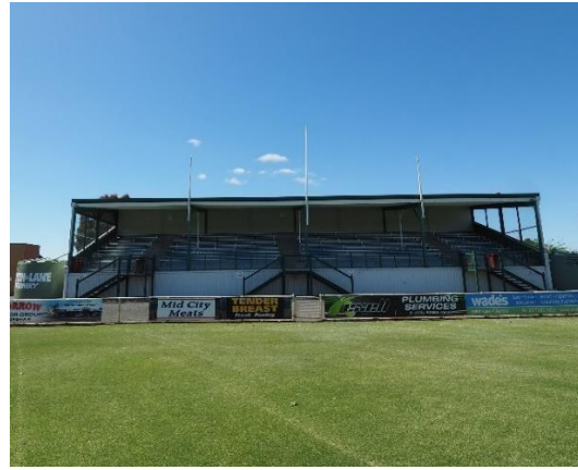
Figures 11, 12: Overall form of grandstand retained: note removal of part of outer stairs, roof platform
