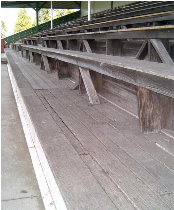
Figures 13, 14: Earlier timber seating and floor finishes, replaced with aluminium bench seats, floors covered
