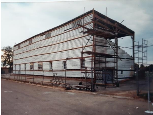
Figure 9: Grandstand prior to recladding:
