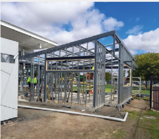
Aquatic Centre frameworks for change rooms.
