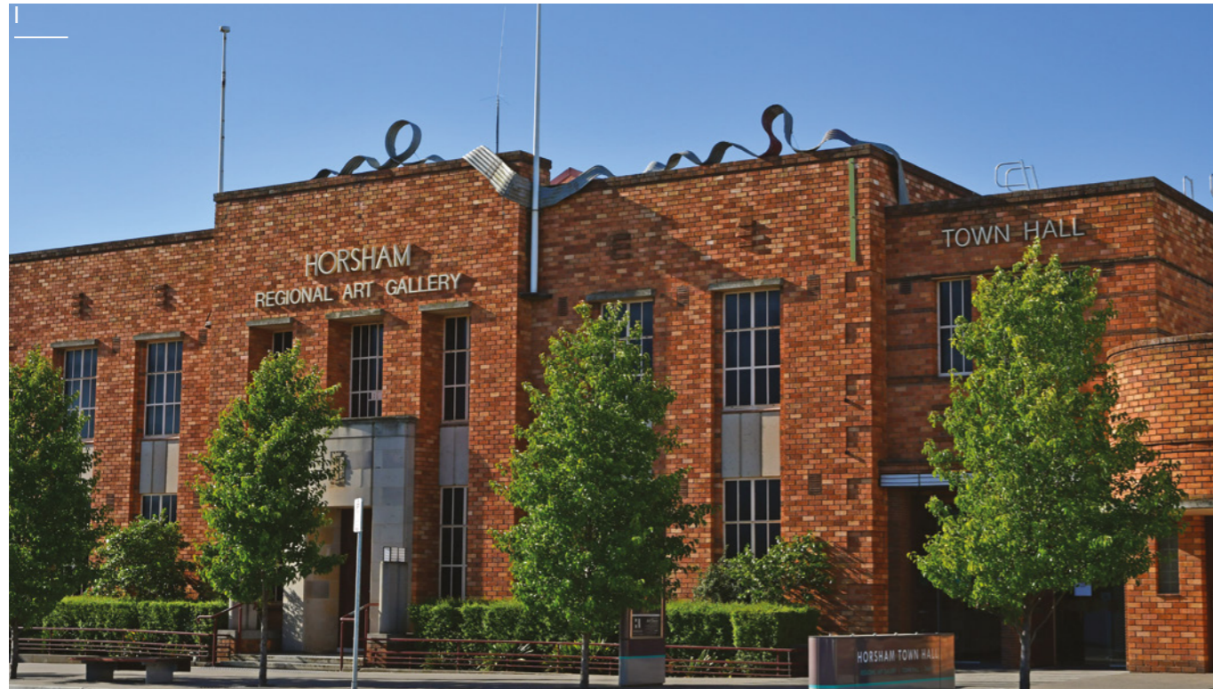
Image: Horsham Regional Art Gallery. Photo: HRCC Archive.
