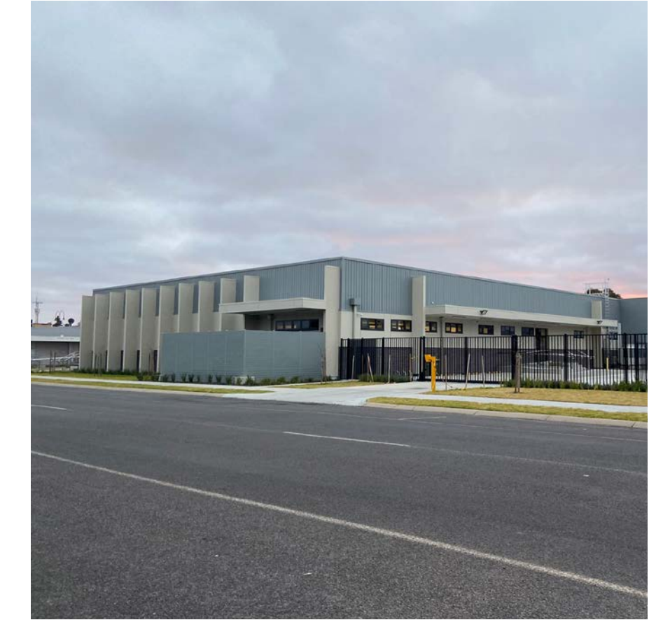
Government Services Building
