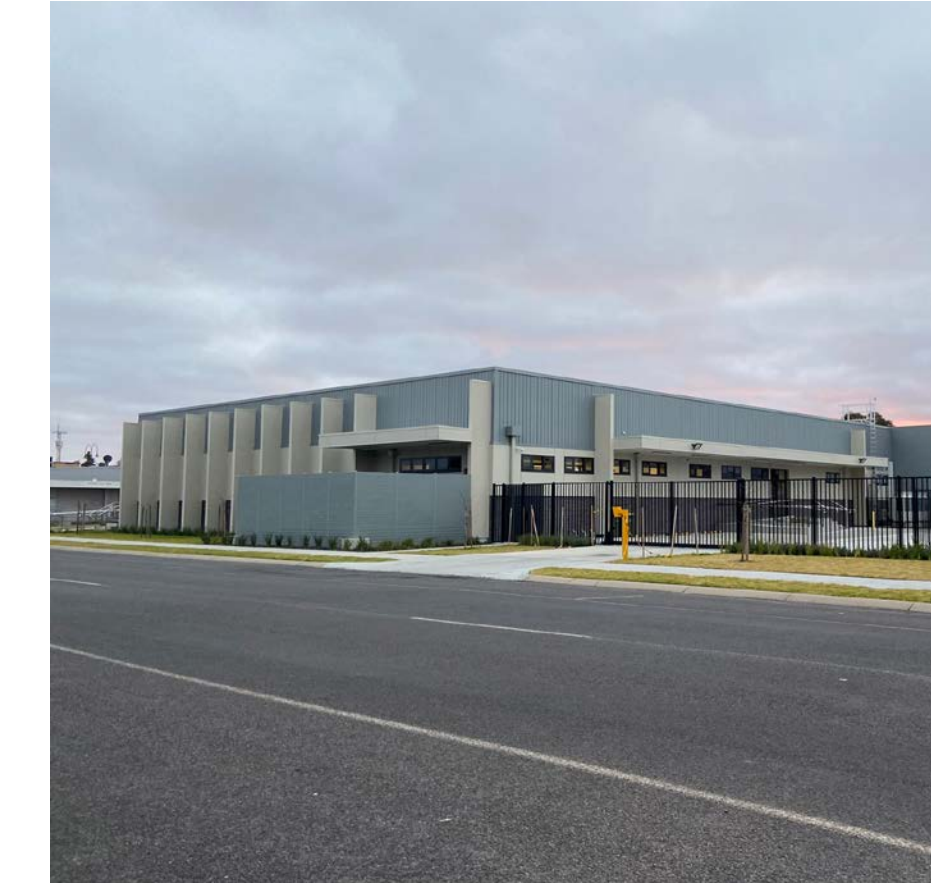
Government Services Building
