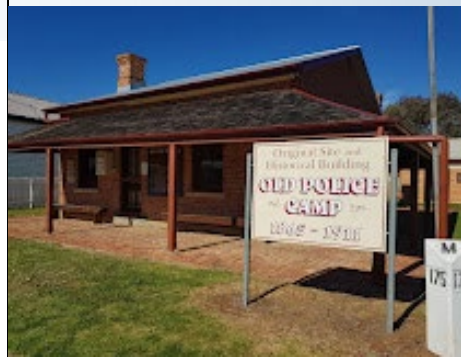
Old Police Station Donald Woods Street, Donald
