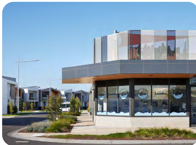
Built form should hug the corners of the street with significant areas of glazing.
