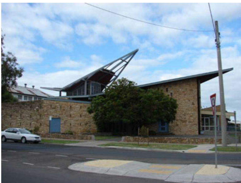
St Andrews Uniting Church, 8 Pynsent Street Horsham 141.JPG
