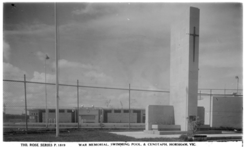
25.2 Horsham Memorial Swimming Pool, opened in 1957 (State Library of Victoria)
