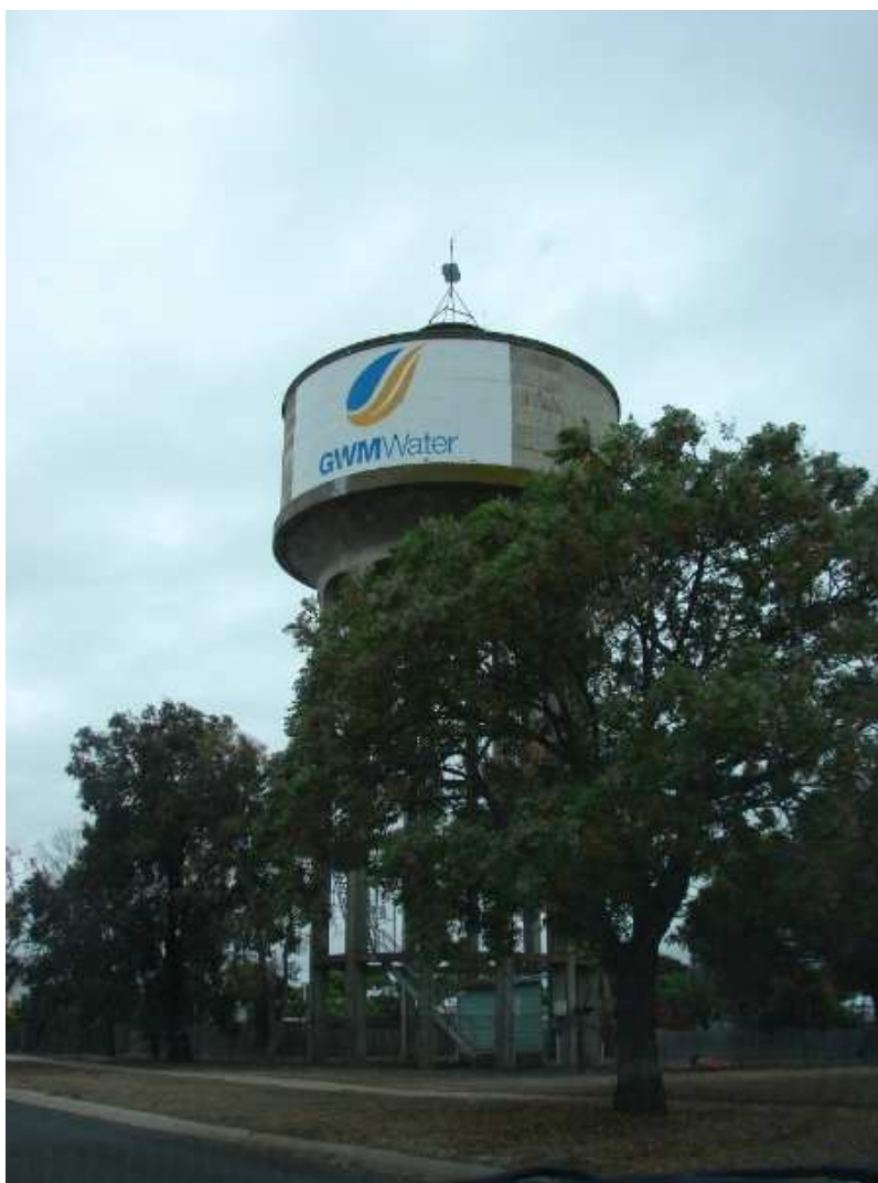
Water Tower, Mill Street corner Gertrude Street Horsham 002.JPG
