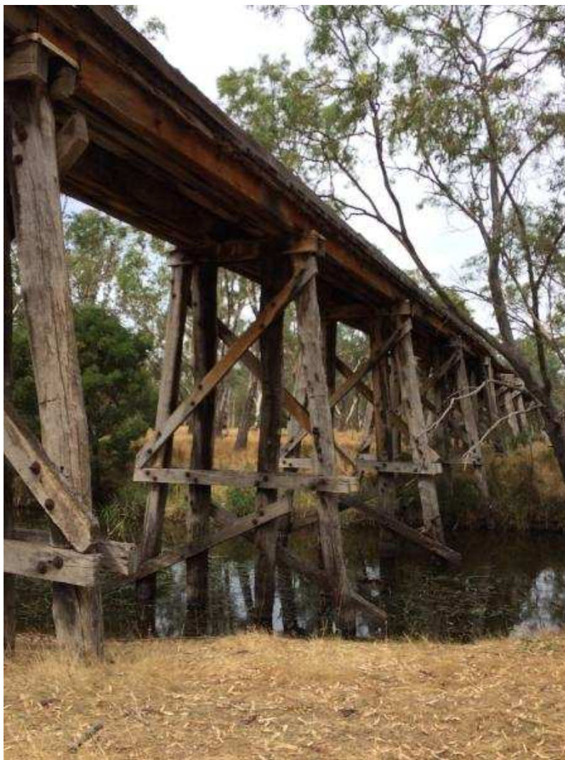
Timber Trestle Railway Bridge over Glenelg River
