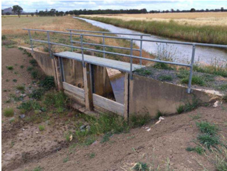
Wimmera Inlet Channel Loop Channel
