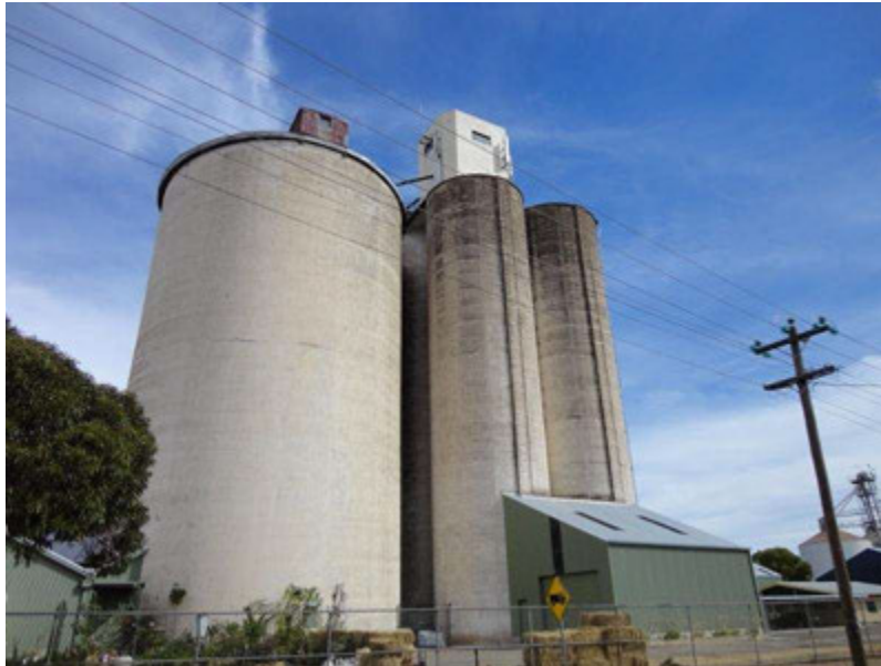
Horsham Silo complex, 35-39 Wawunna Road Horsham.jpg
