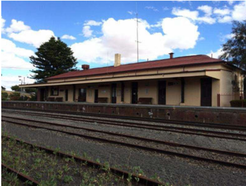
Horsham Railway Station and Goodshed, Railway Avenue Horsham
