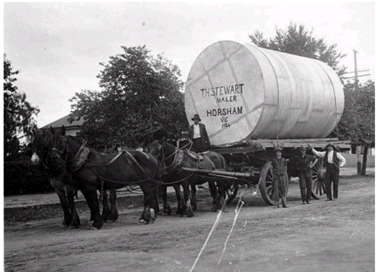
23.1 Horse-drawn dray delivering a water tank manufactured in Horsham, 1924 (State Library of Victoria)
