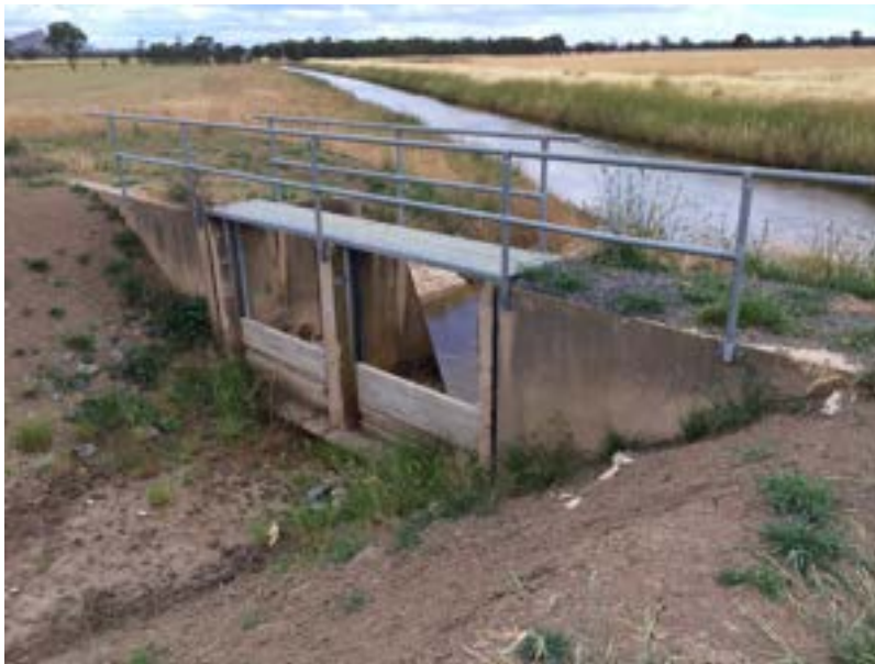
Wimmera Inlet Channel Loop Channel
