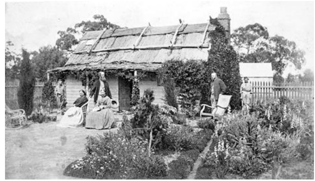
9.3 timber cottage at Green Park, near Horsham, with characteristic bark roof, c.1875 (Museum of Victoria)
