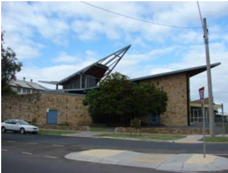
St Andrews Uniting Church, 10 Pynsent Street Horsham
