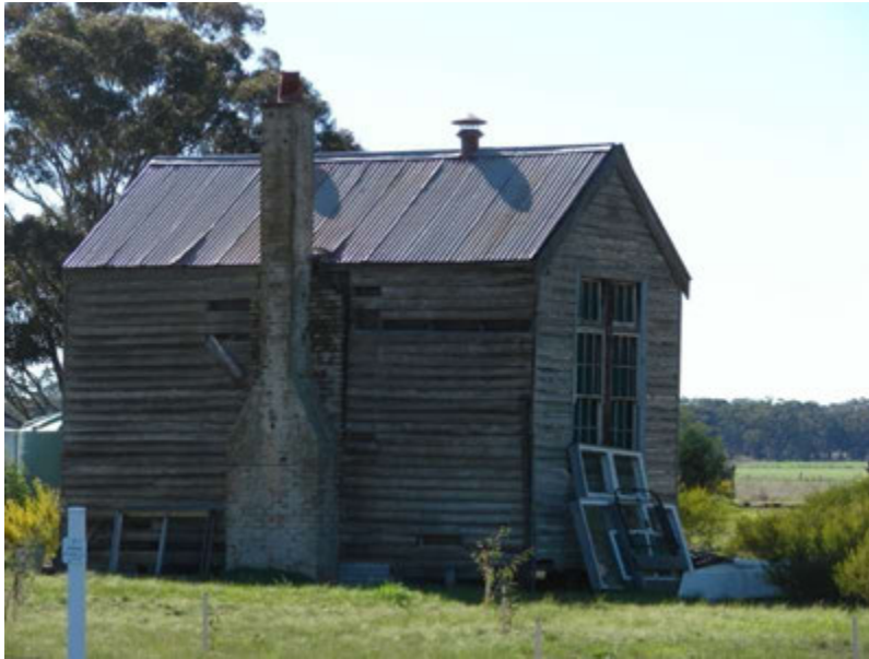
Former Polkemmet State School, 196 Polkemmet East School Road, Pimpinio DSC08016.JPG
