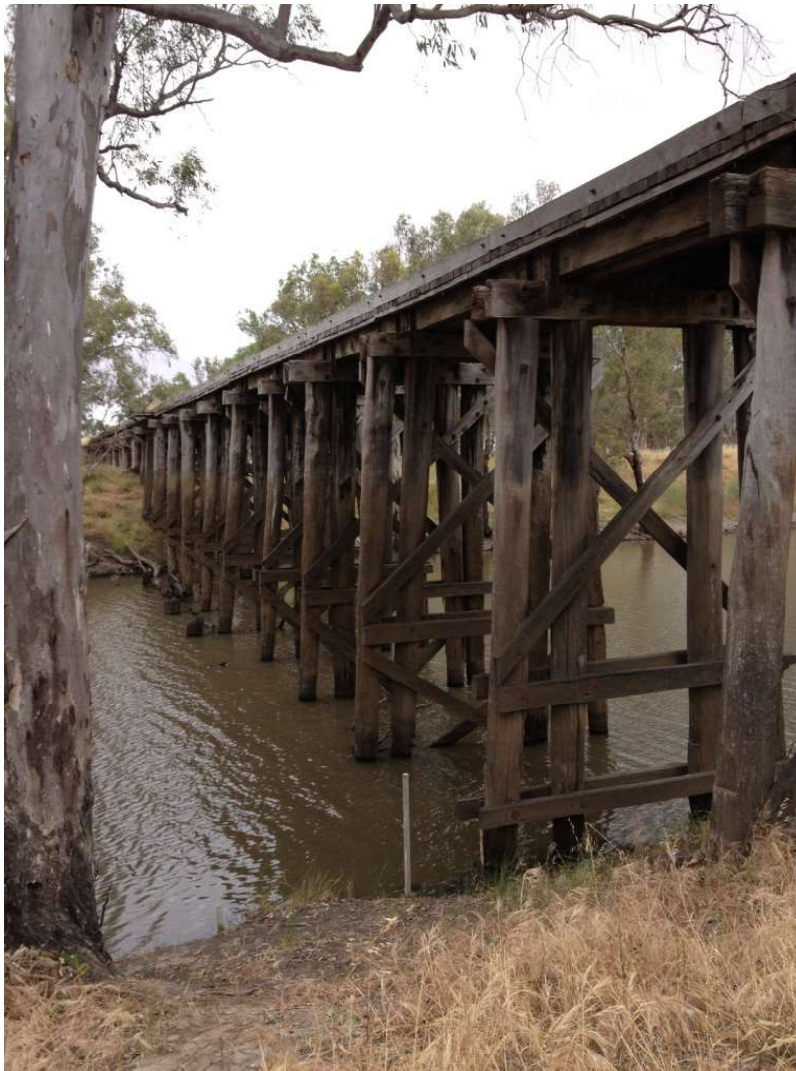
Timber Trestle Bridge over Wimmera River at Quantong
