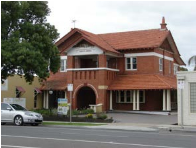
'Droylsden', 143-145 Baillie Street Horsham
