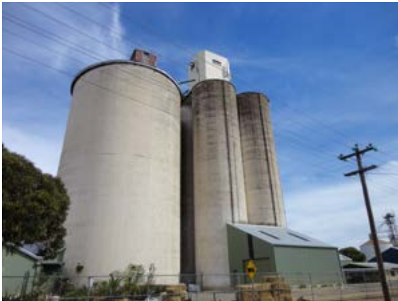
Horsham Silo complex, 35-39 Wawunna Road Horsham
