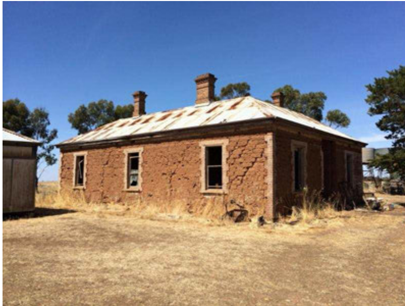
Oakville Park homestead complex, Vectis Station Road Vectis
