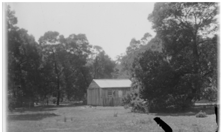
11.1 Timber bee-keeper's hut belonging to Matthew Matthews at Bald Hills, Laharum (State Library of Victoria)
