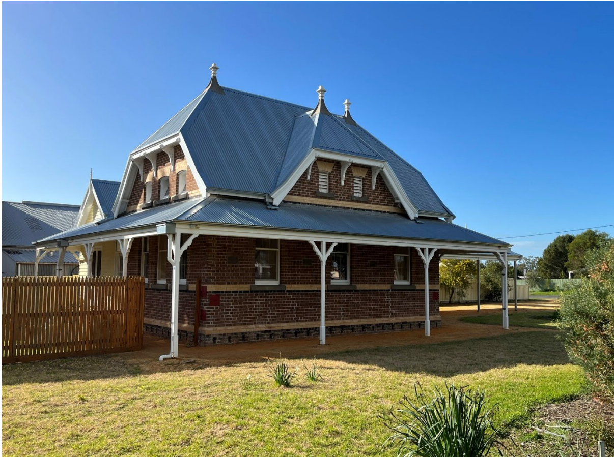
Former Natimuk State School, 1a Sudholz Street, Natimuk, viewed from Main Street (GGA, September 2023)
