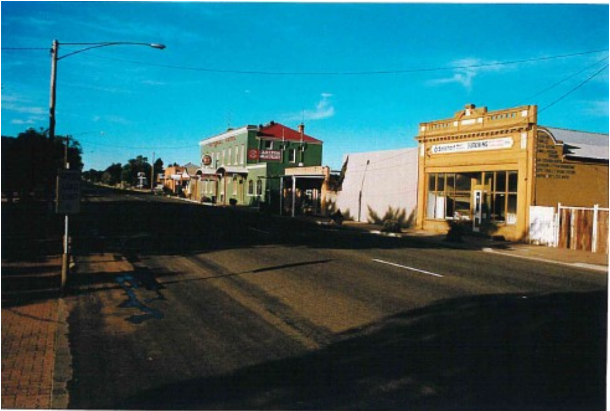
Main Street overlooking east from Schurmann's Shop, Natimuk Historic Area
