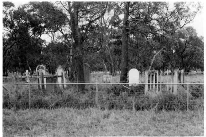
7.4 The former Polkemmet station cemetery dates to 1860, photographed in 1979 by John Collins (State Library of Victoria) little remains in 2014 – only broken headstones.
