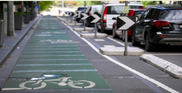
Protected cycle lane – Physical barrier and signage separates cycling from other road use.
