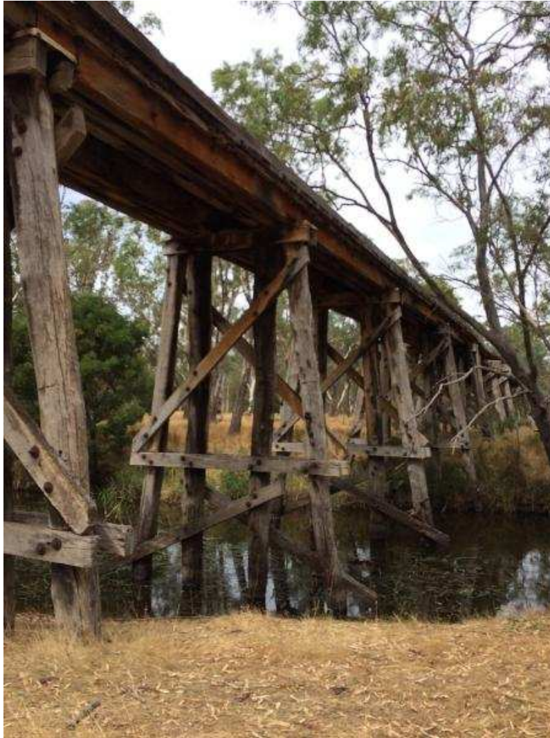
Timber Trestle Railway Bridge over Glenelg River
