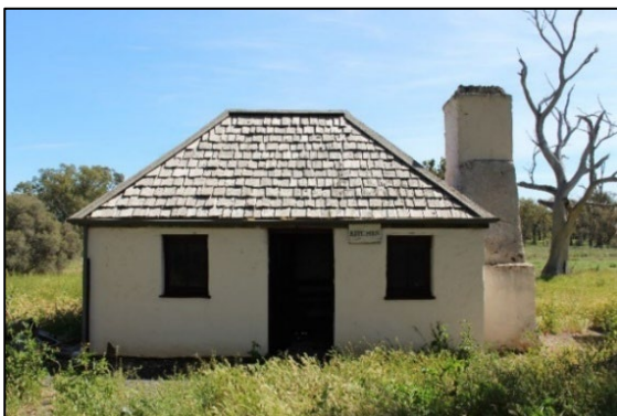
Photograph 7 Kitchen at Ebenezer Mission, 24 October 2017
