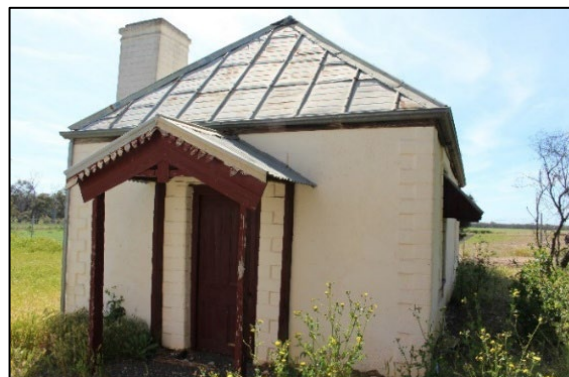
Photograph 8 Dormitory at Ebenezer Mission, 24 October 2017
