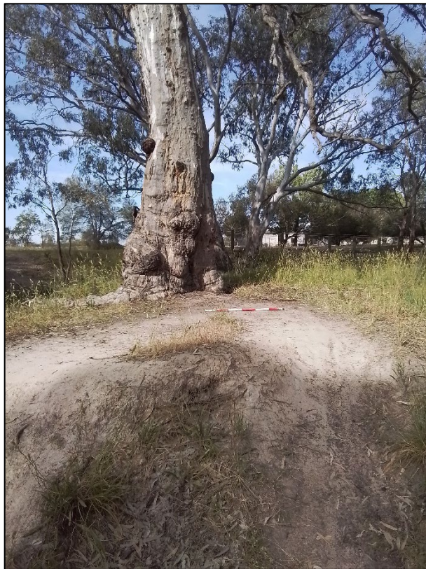
Photograph 14 Looking south-west across eroded turn around point along bike track, 12 December 2025
