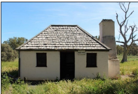
Photograph 7 Kitchen at Ebenezer Mission, 24 October 2017
