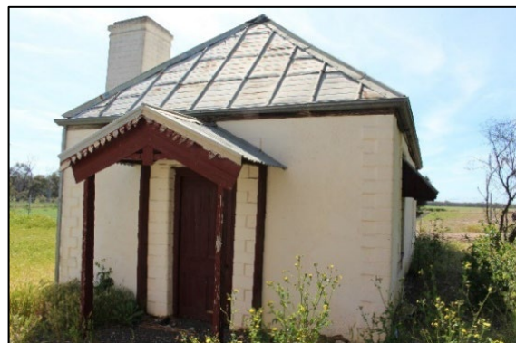
Photograph 8 Dormitory at Ebenezer Mission, 24 October 2017
