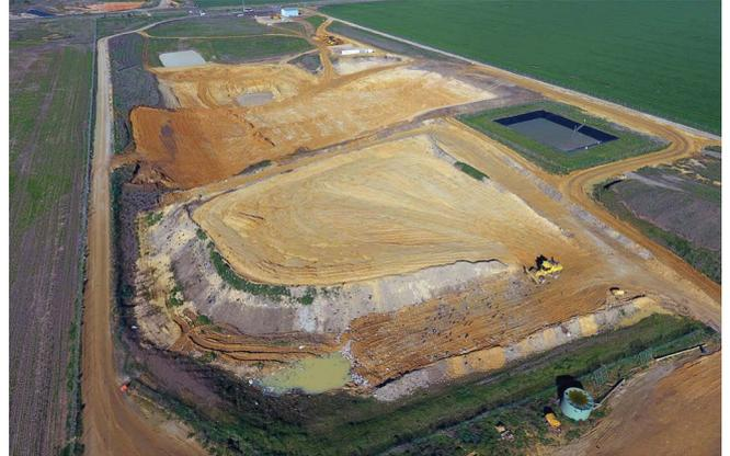
The landfill site showing the current cell approaching capacity in the foreground, with the new cell under construction in the background
