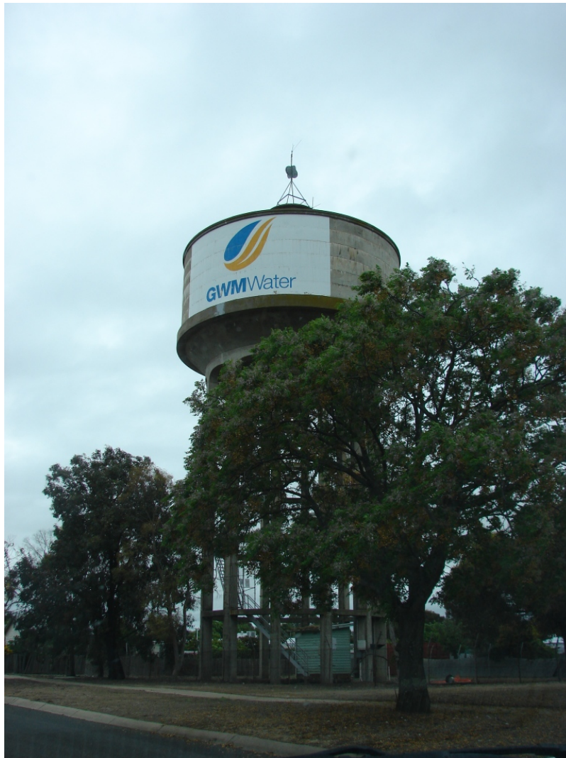
Water Tower, Mill Street corner Gertrude Street Horsham
